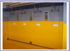
All areas were washed, cleaned, and acid etched to remove glazing. After masking, 251 Primer was applied followed by Duraspray. Top Coat was then applied along with aggregate for its non slip properties.
